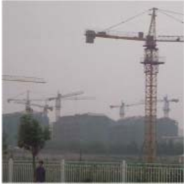
Picture 2 – Cranes in Chengdu
