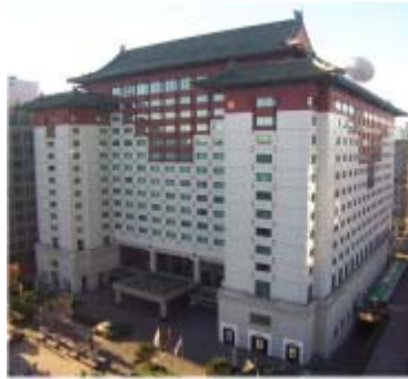
Picture 1 - New/Modern Blend Construction
